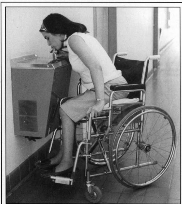
One of the early redesigns of a drinking fountain, changing the location of the spigot and control, with a receding front wall, so that people standing or sitting could enjoy a cool drink was a part of the U of I research in the 1950s.
