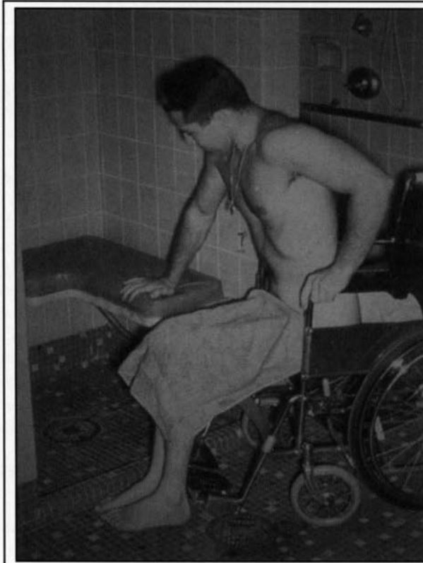
A seat, designed to give a person with paraplegia or quadriplegia a safe secure setting in which to take a shower, was built to fold flat against the wall to give an able-bodied person room.
